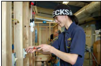
Above: George Kameroff works on wiring a mock-up wall during Residential Electrical.
